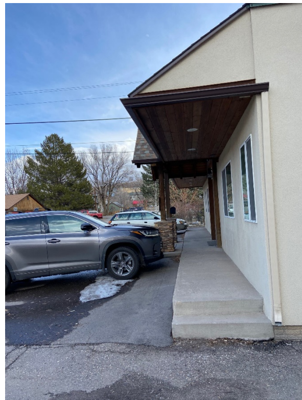
Figure 3 – West, looking East – sidewalk and entry encroachment
