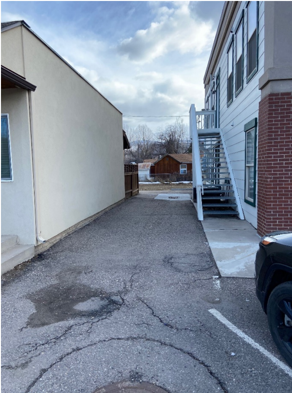
Figure 4 – Driveway between 404 Broadway & 113 E. Fourth St. (property of 404 Broadway)
