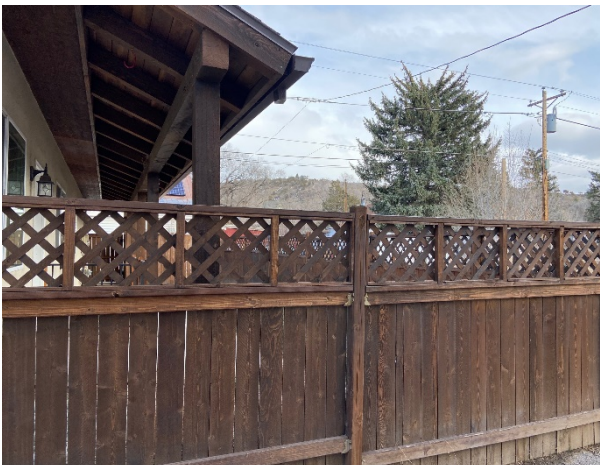
Figure 6 – Rear fenced area – West side of building looking East
