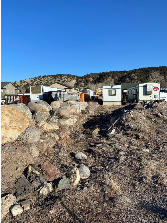
Figure 8 - Southwest corner looking North
