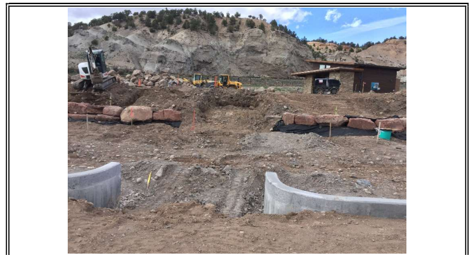
Beach Sand Area and Stair Case Rough Grading
