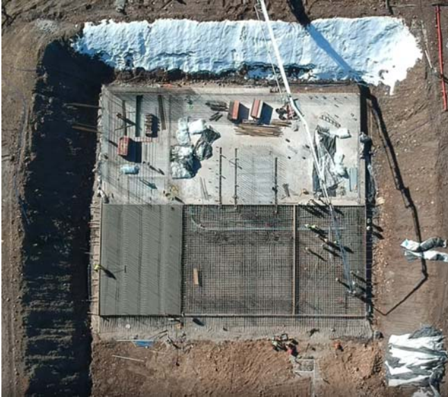
Aerial Photo of Treatment Building Structure 3/20/19
