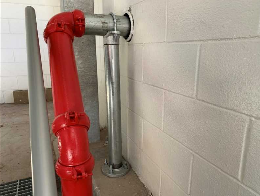
Stand Pipe for Fire Dept. Installed
