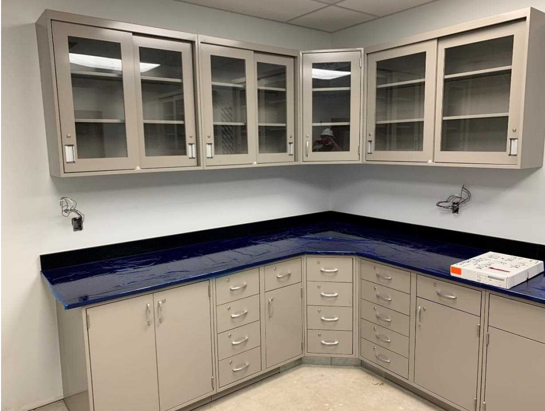
Lab Cabinetry Installed
