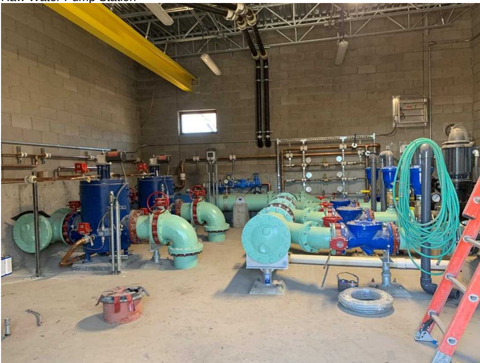
Raw Water Pump Station
