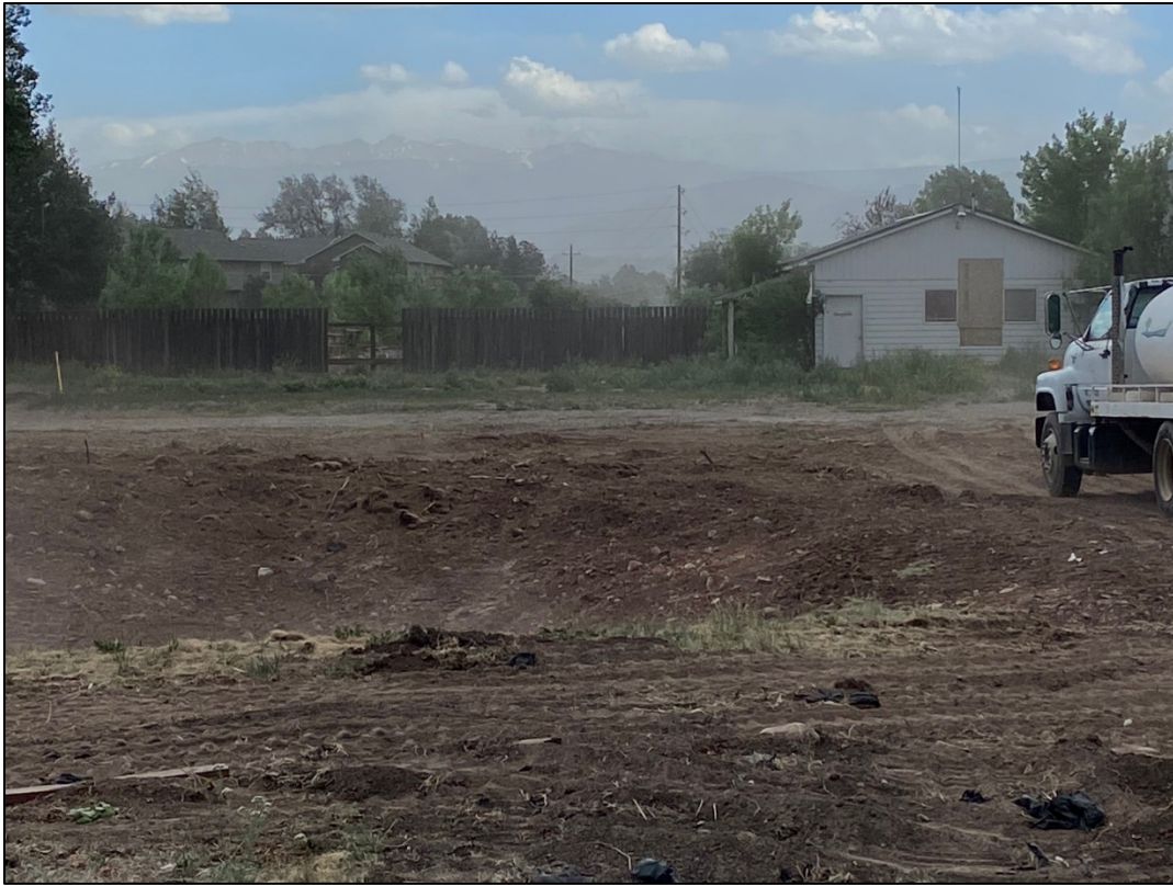
762 & 768 Castle Drive and the rear alley
