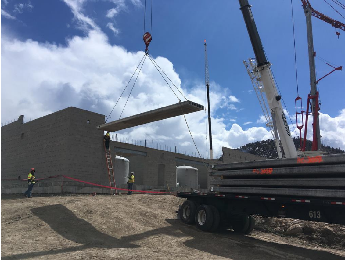
Set Precast Roof Panels 3-30-20
