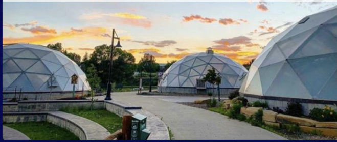
Geothermal greenhouses – Pagosa Springs
