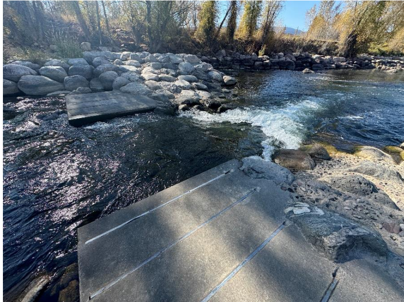
Figure 2: Existing conditions at Drop 2 showing concrete pads, grouted rock wings, and end of island. Image captured by REP during the site visit.
