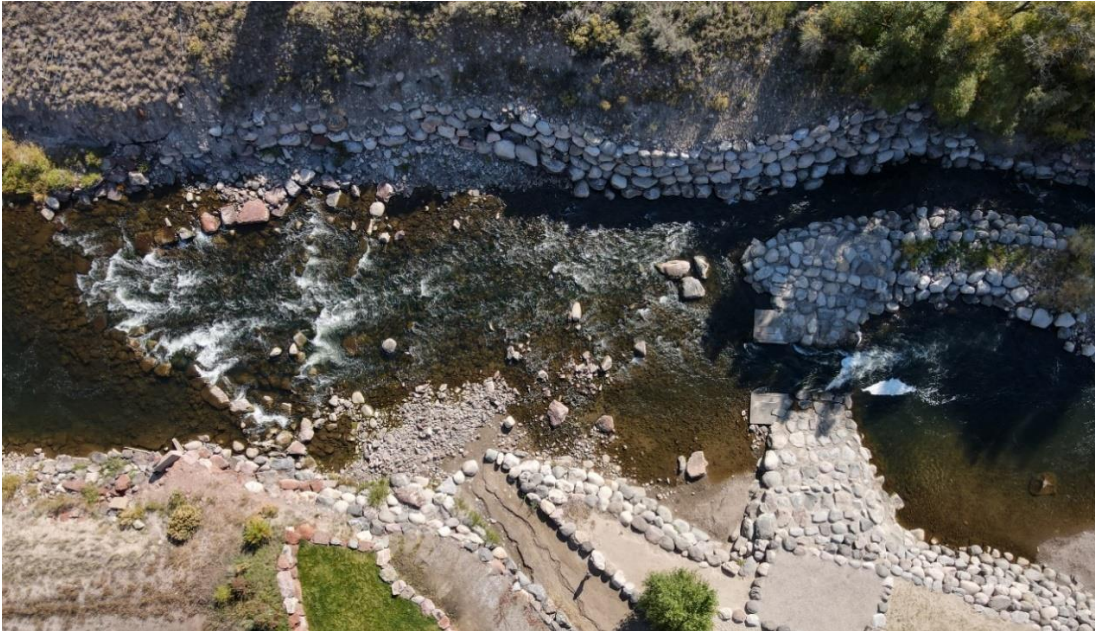
Figure 3: Drone photo captured during REP site visit of the existing diversion structure, rock riffle, and Drop 1.
