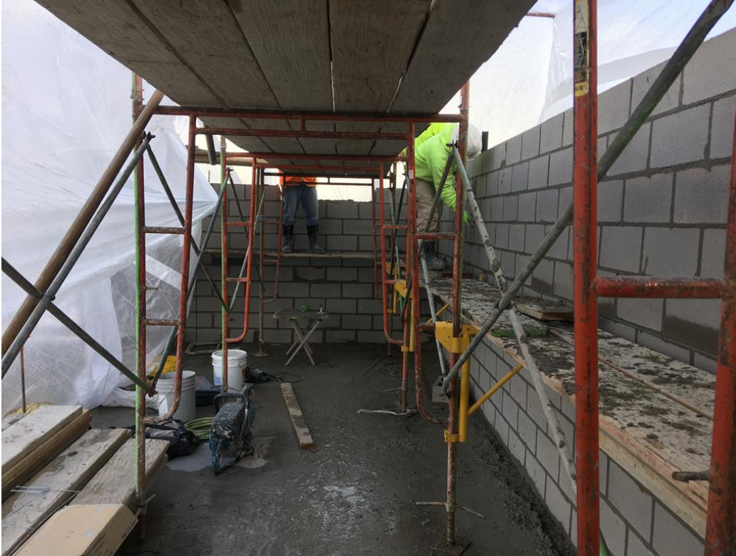
Structural Masonry Install 2-05-20
