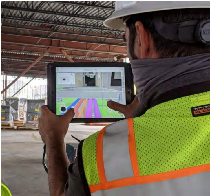
A JHL superintendent uses Procore to inspect work and confirm it meets expectations.
