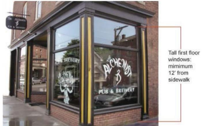
Figure 4.10-E: First floor window height
