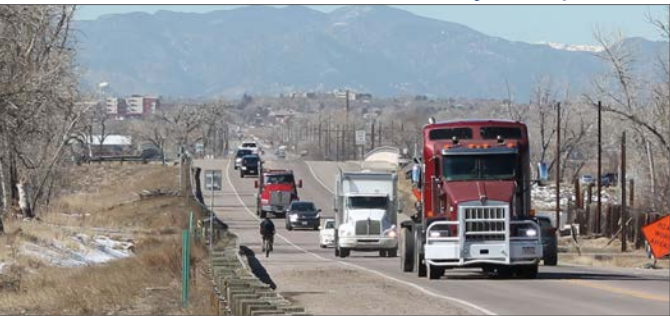
104 Avenue Widening - Thornton, CO
