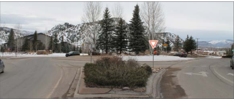
Sylvan Lake Rd Roundabout - Eagle, CO
