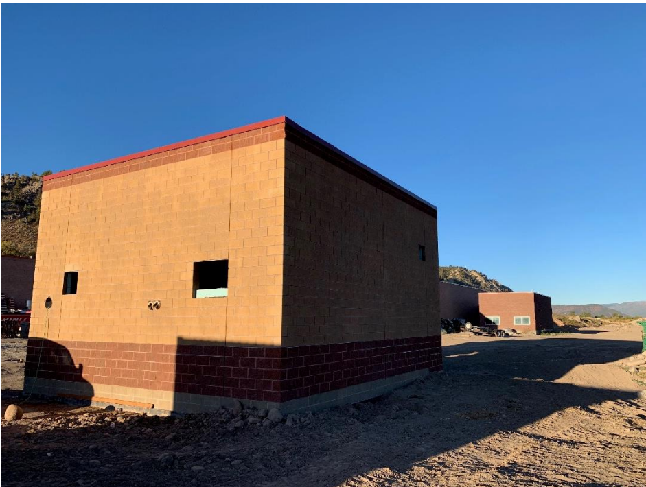
RWPS Roof Done 10/1
