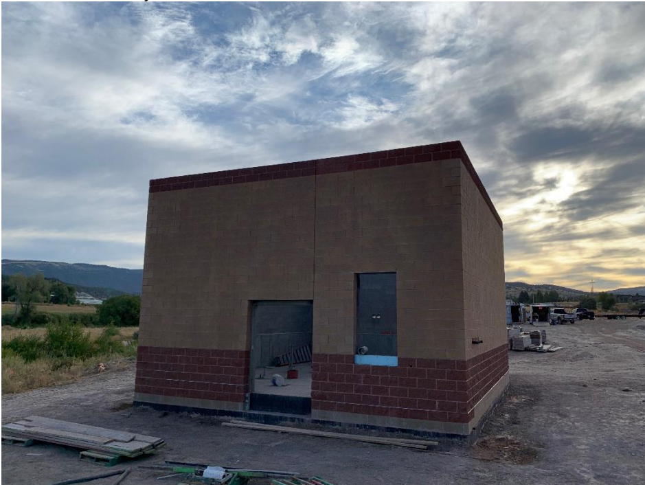
RWPS with Masonry Veneer 9/3
