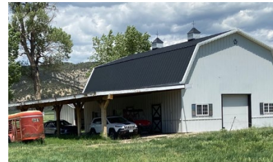
Brush Creek Rd – Vertical Siding
