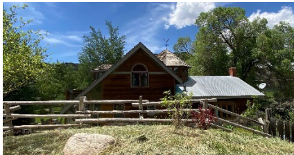
Brush Creek Rd – Wood Siding
