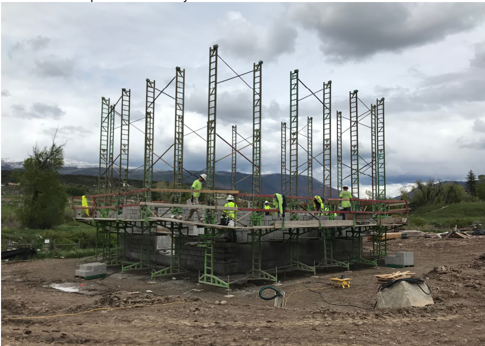
Raw Water Pump Station Masonry 5/29/19
