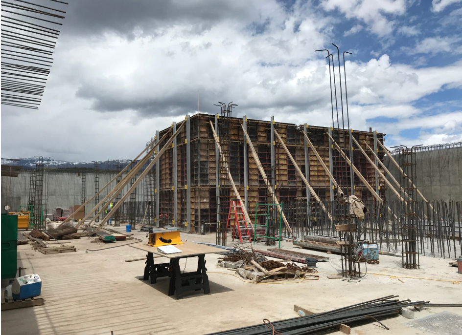
Treatment Building Interior Structure 5/29/19
