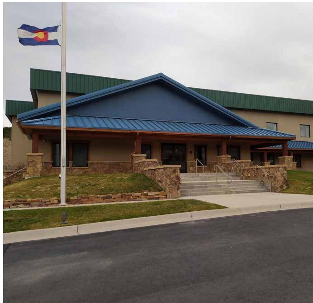
Chambers Ave Commercial Building
