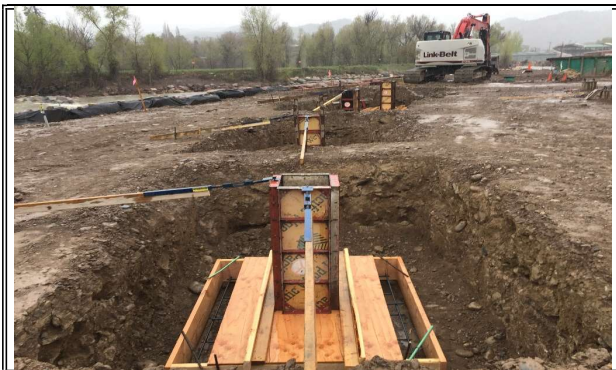
Pavilion Structure Foundations
