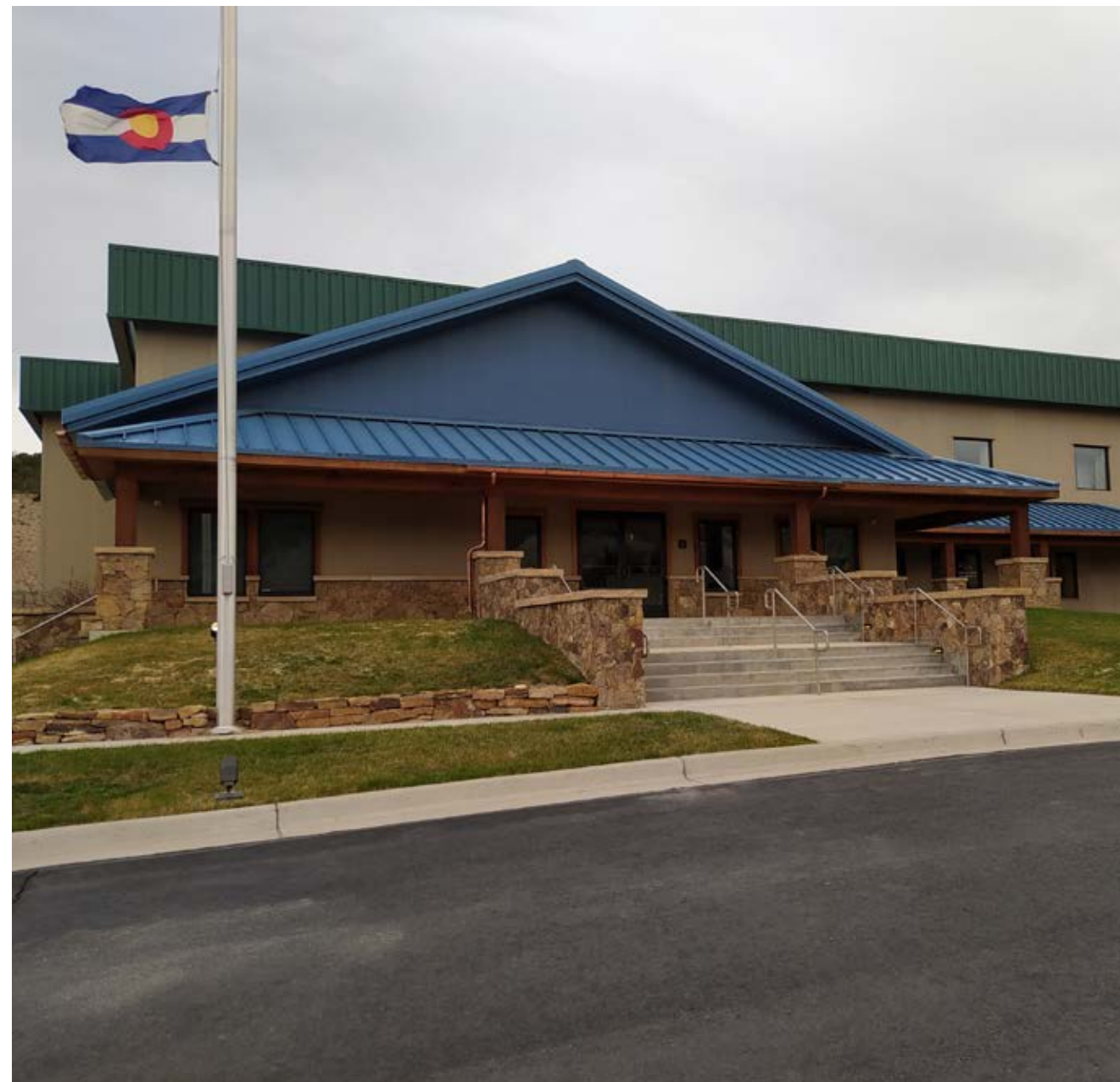
Chambers Ave Commercial Building
