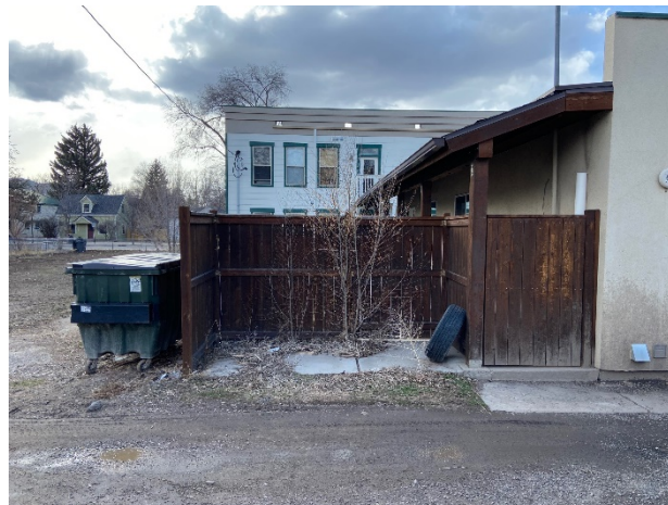
Figure 7 – Rear fenced area – East side of building looking West
