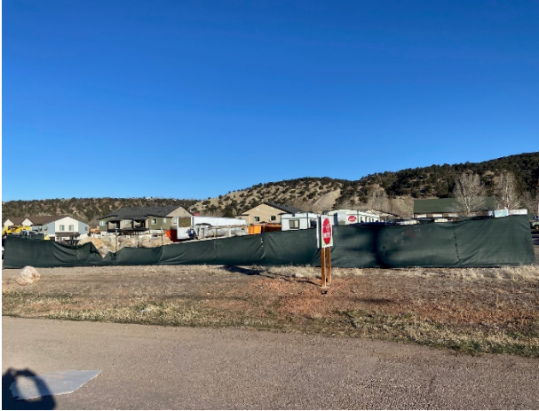
Figure 4 - North from Sawatch Rd towards 629 Sawatch
