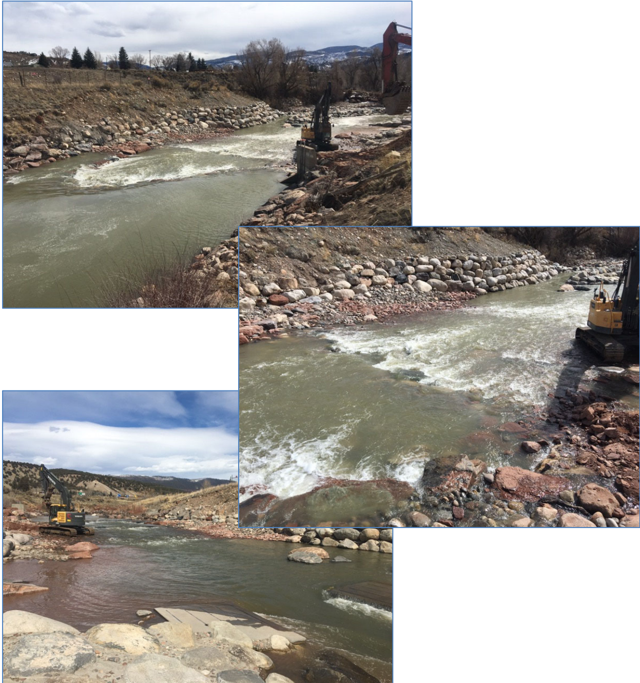
Figure 6: Completed Diversion Structure & Riffle Reconstruction
