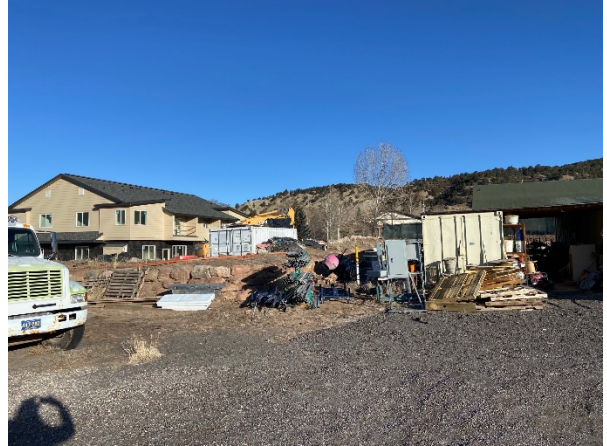
Figure 9 - from 629 Sawatch looking towards 700 Chambers, Building D
