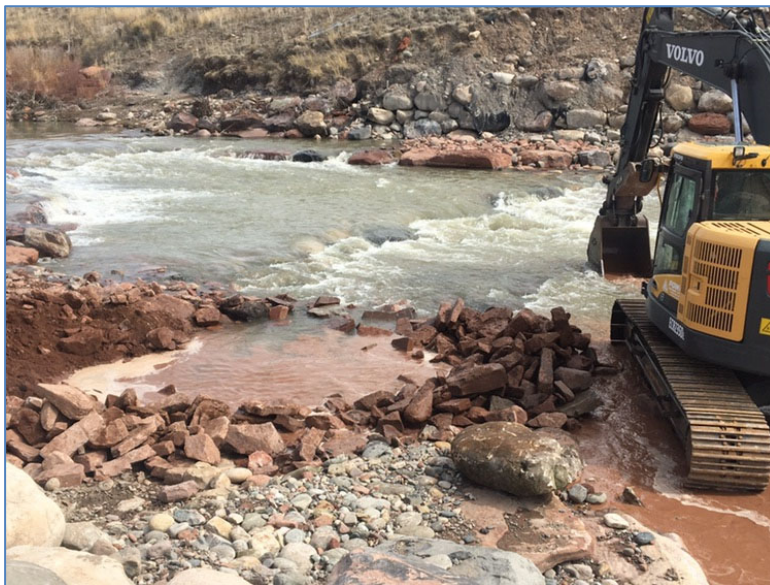
Figure 5: Hobbs Packing Angular Material in Between Grade Controls
